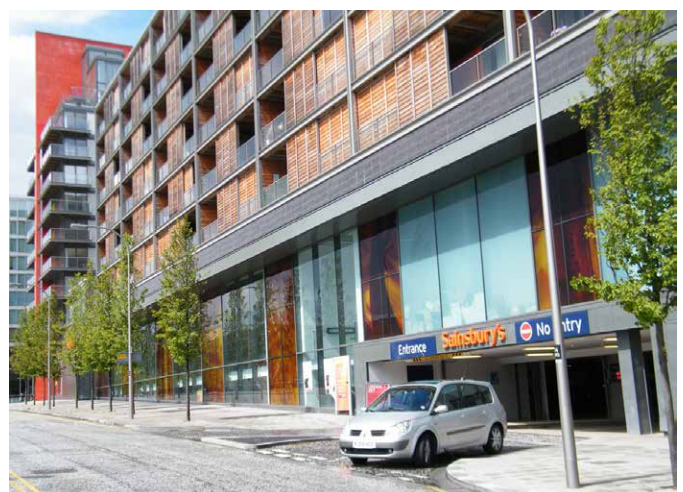
Example of an integrated parking solution (Vizion Development, CMK) where the car park entrance is kept to a minimum and designed as part of building facade
