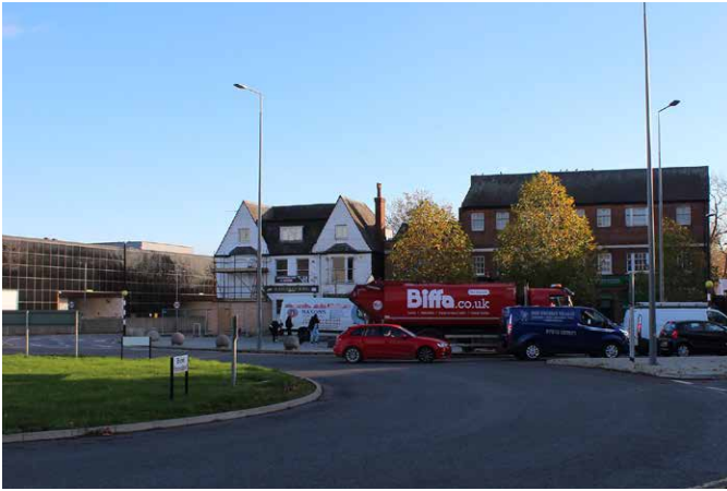
The area fronting onto Brunel Roundabout comprising Victorian buildings and back of The Brunel Shopping Centre
