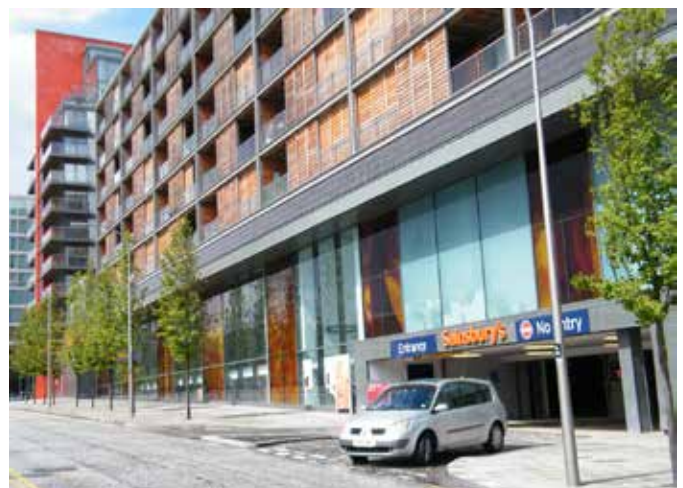
Example of an integrated parking solution (Vizion Development, CMK) where the car park entrance is kept to a minimum and designed as part of building facade
